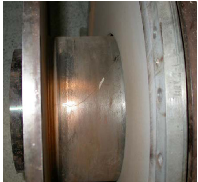
Figure 1: Failed coupling (spacer crack)
