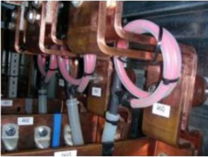
Figure 4: Current probes installed on VSDS links
