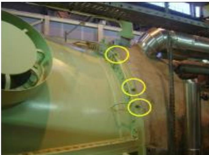
**Figure 3:** Position of 3 sensors on the turbine exhaust casing
