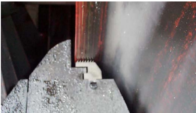
Figure 14. Polymer eye seal in DuPont charge gas compressor after 5 year run.
