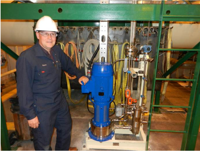
Figure 28: Installed centrifugal booster skid
