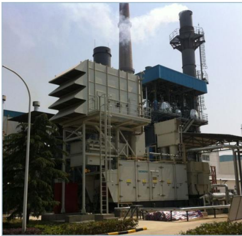
Figure 19: Gas turbine operating on weak gaseous fuel (photo courtesy of Siemens)
